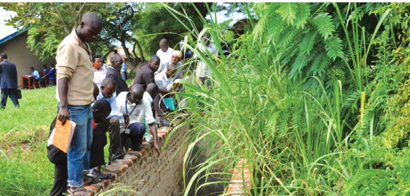
Figure 3: Karugutu Monitors inspecting a latrine under construction at Karugutu SSS
