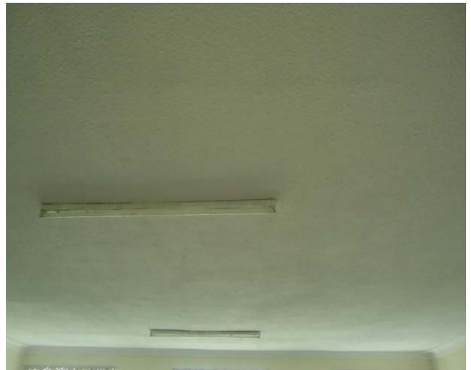
Ceiling fixed after Monitors' intervention
