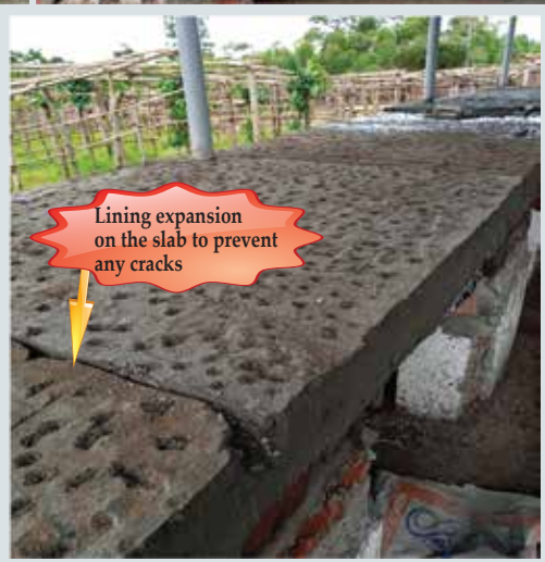
Slab being reconstructed
