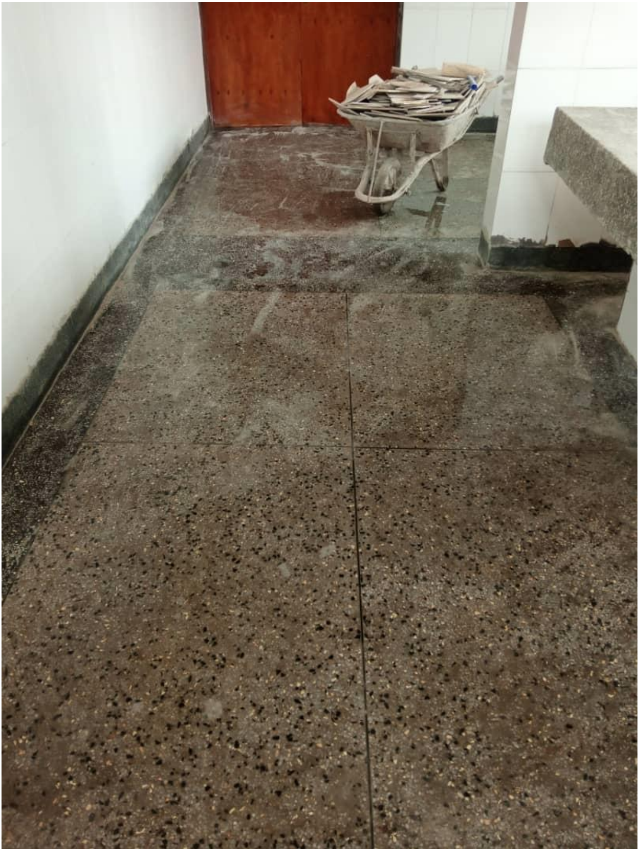
Figure 9: Tiles being removed and replaced by terrazo
