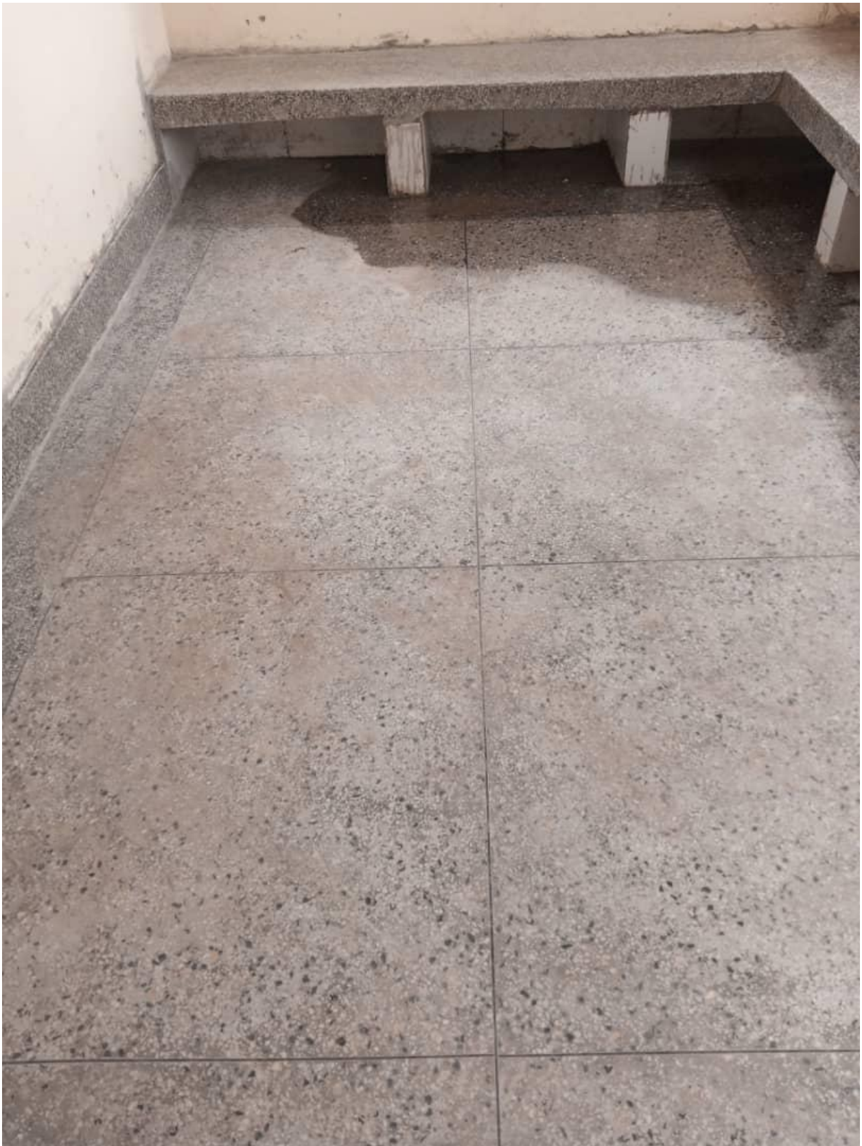
Figure 10: Mortuary floor with new terrazo
