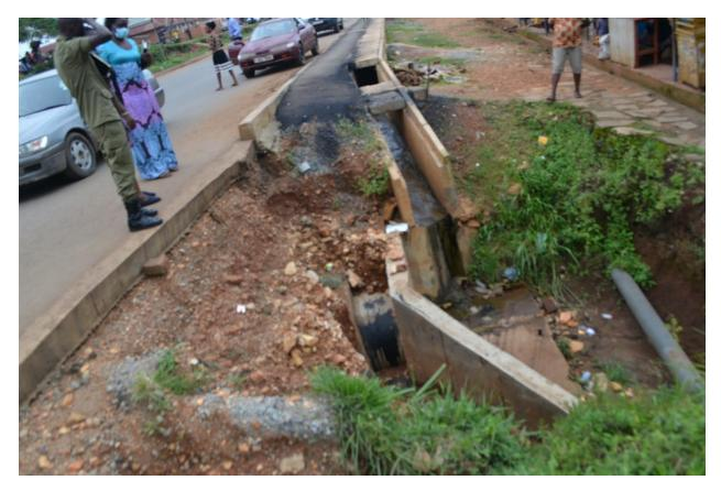
Figure 10: Poor drainage system in Karambi - North Division Fort Portal
